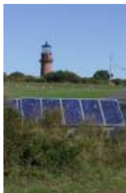
This 1.6-kW PV array, which supplies green electrons to a public restroom in Aquinnah, is one of many systems that are helping reduce the Vineyard’s dependence on energy from the mainland.
