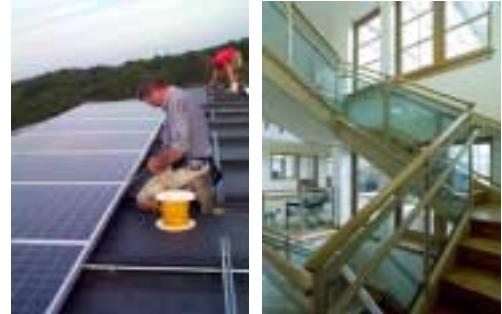
In green buildings, active and passive solar energy solutions, including rooftop PVs and daylighting, reduce demands for energy from off-site sources. (credit: WHRC)
