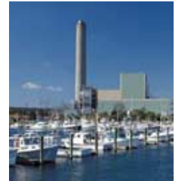
The Canal Station burns fuel oil to supply most of the electricity consumed in the Cape & Islands region. (credit: Mirant)
